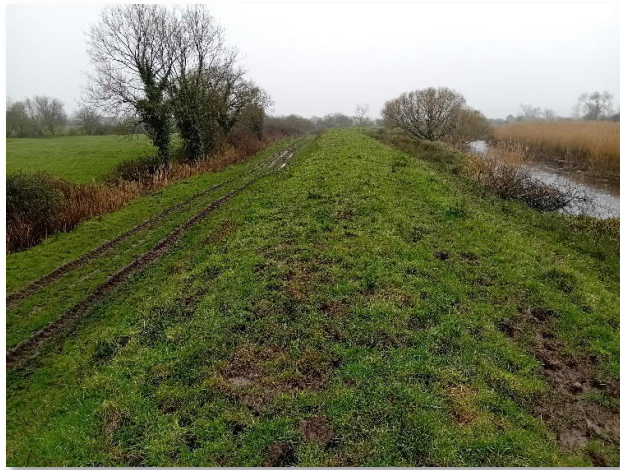
Image 4-9: E9 – Poached / rutted GA1 on embankment footprint and fringing areas
