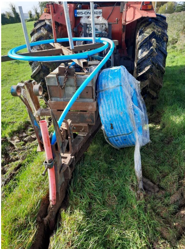
Plate 10: Installation of drinking water supply via mole.
