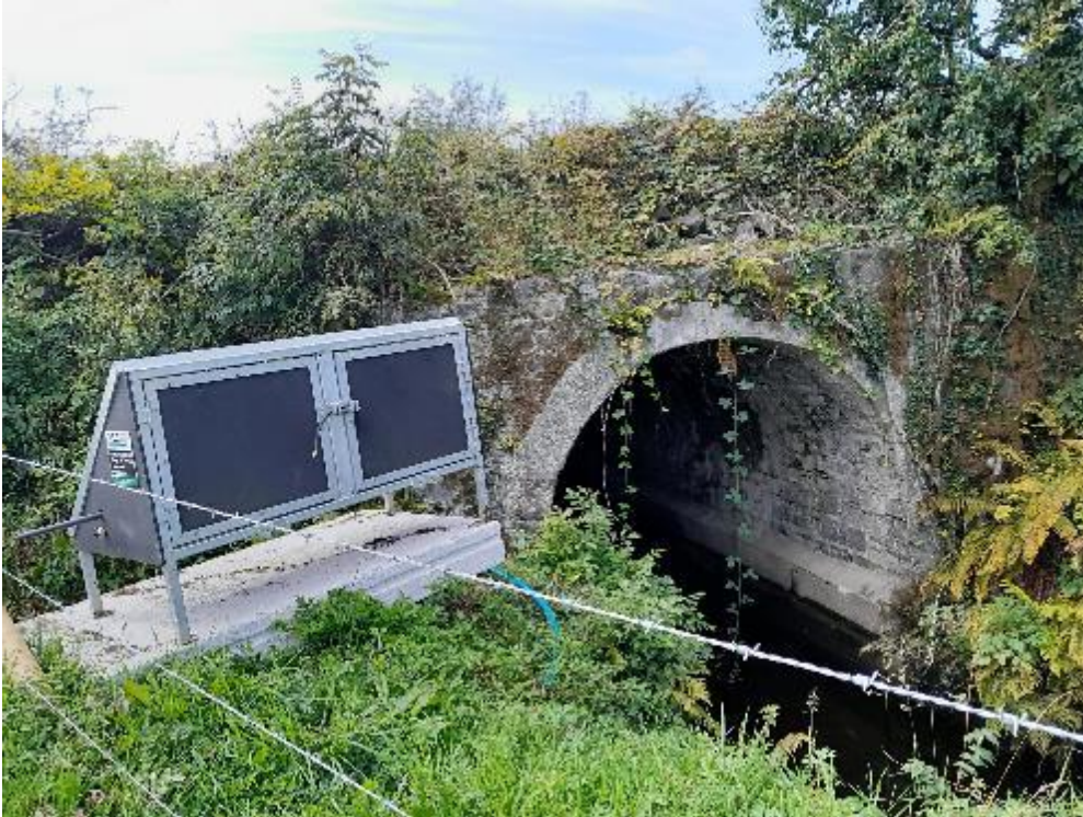
Plate 1: Double panel solar pump on the Mountnugent River
