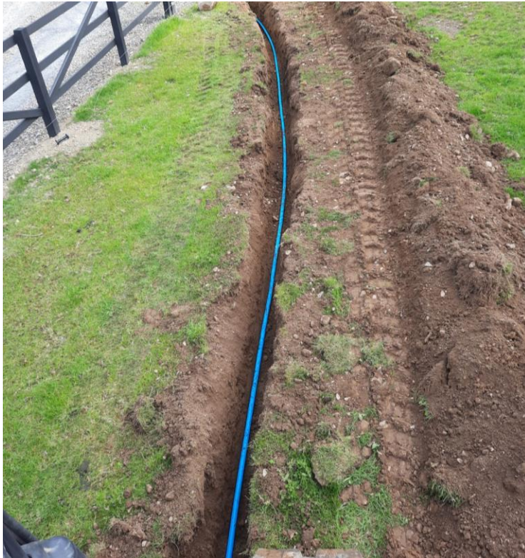
Plate 11: Installation of drinking water supply by cut and cover method.
