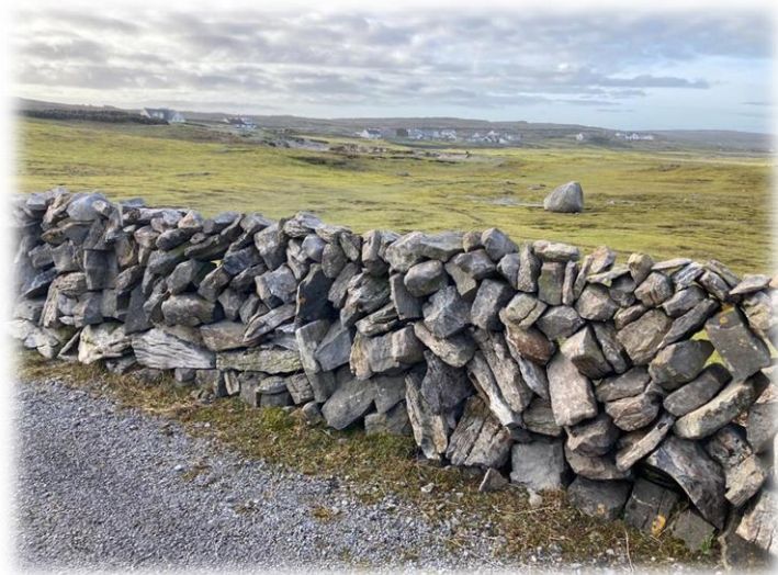
Fig.17 Part of the stone wall built on the east side of the Machair to control grazing and reduce access to vehicles.
