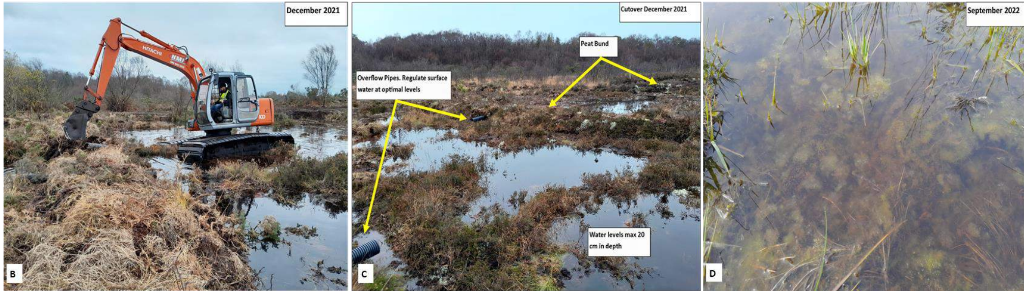
Plates 4.2 (a) (b) and (c): Overflow pipes were adjusted to regulate surface water levels at optimal levels for Sphagnum establishment on the cutover in December 2021 (A); peat bunds were constructed into compartments to hold water on the cutover at depths of 20 cm (B); and the establishment of pioneer Sphagnum mosses (Sphagnum cuspidatum) in rewetted sections of the cutover monitored during September 2022, 10 months after rewetting was completed (C).
