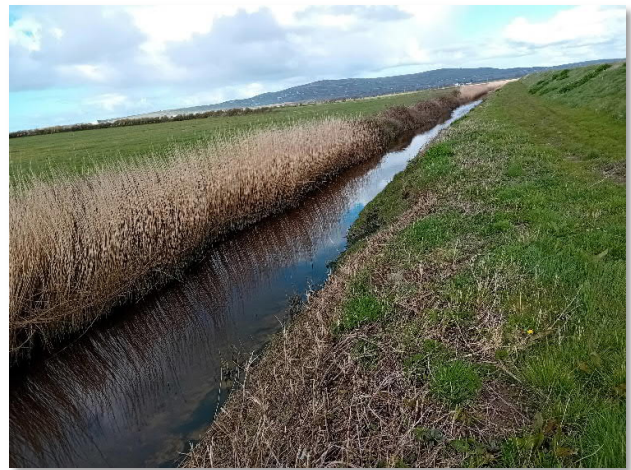
Image 4-4: Back drain fringing the embankment infrastructure
