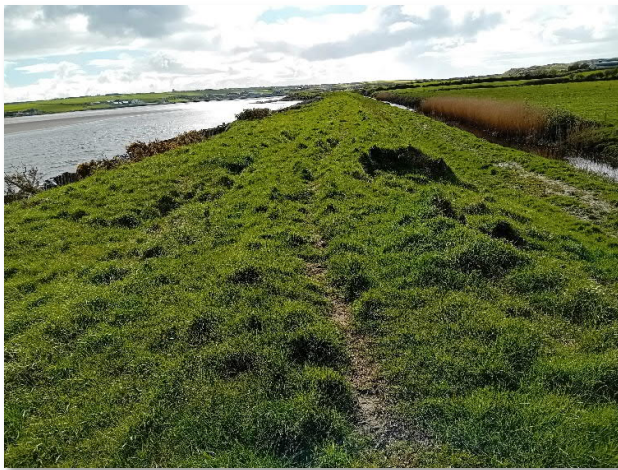
Image 4-3: In-situ grassland at the crest of the embankment
