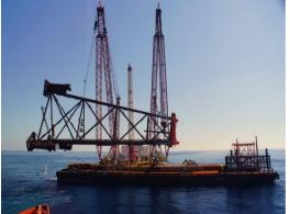
Removal of platform jacket onto barge for transport to shore
