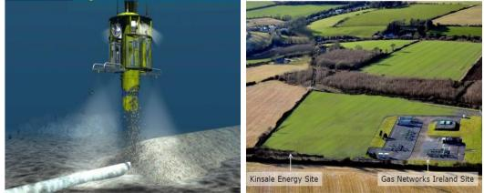
Rock placement along exposed pipeline
