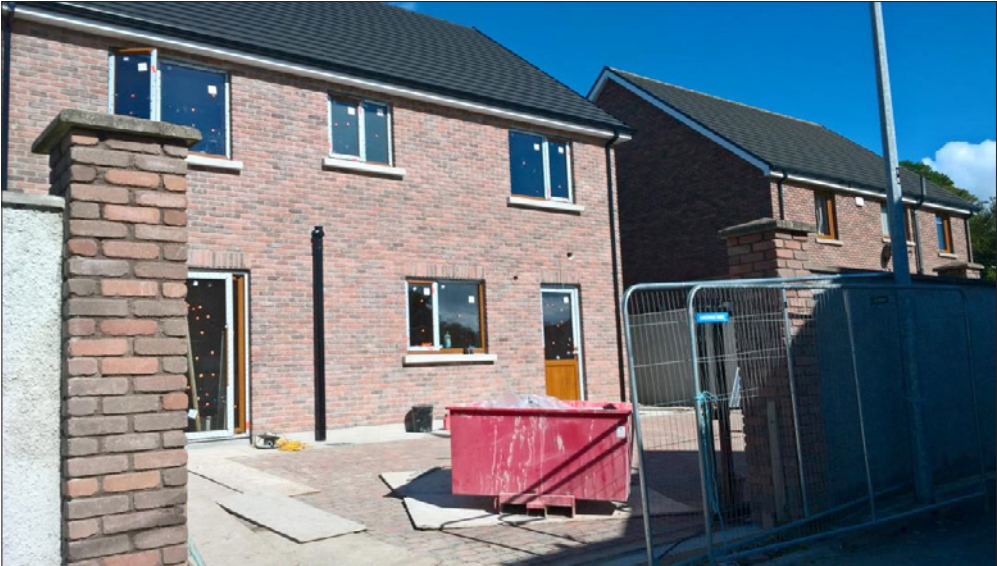
Active construction site – units facing main road
