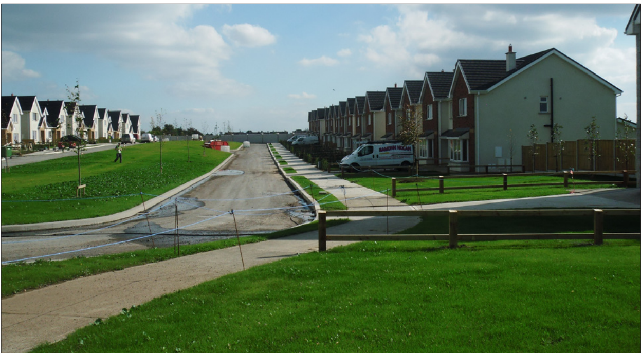
Completion works - Fruithill Manor, Graigecullen, Laois
