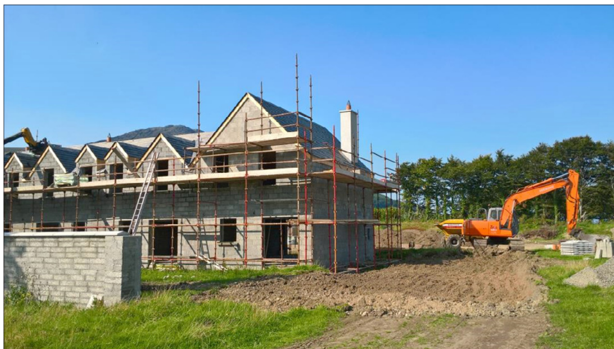
Active construction site
